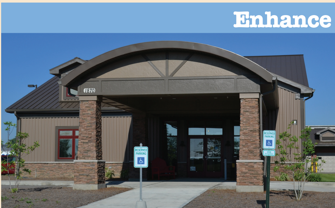
HCSS and HART now reside on 1.67 acres on Fields Boulevard equipped with a 14-bay garage and 4,000 square feet of office space.
